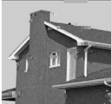
(g). The reconstructed House using UVLC
